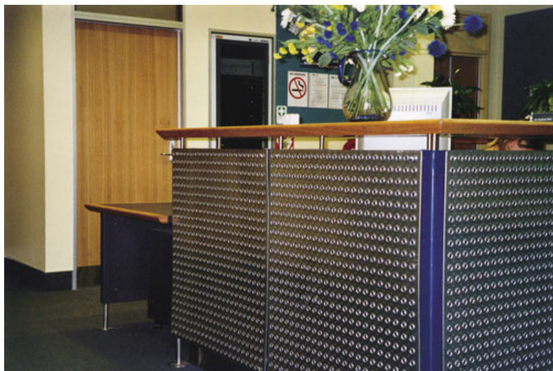
A high reception counter with the accessible section around the corner and not visible on entering.
