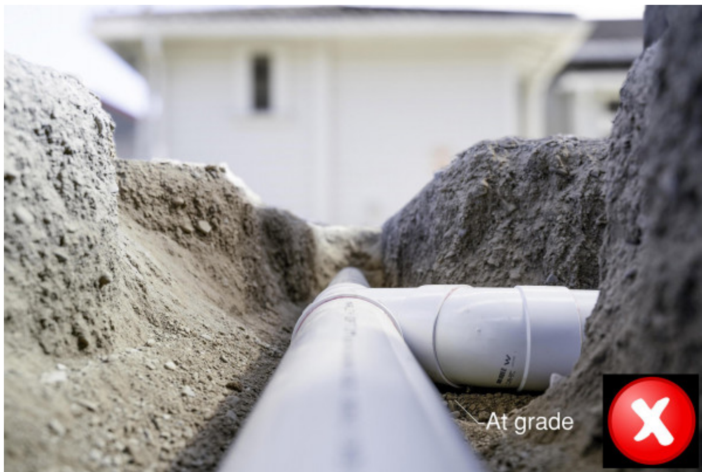
DN100 drain with 45° 'Y' junction installed at grade.
