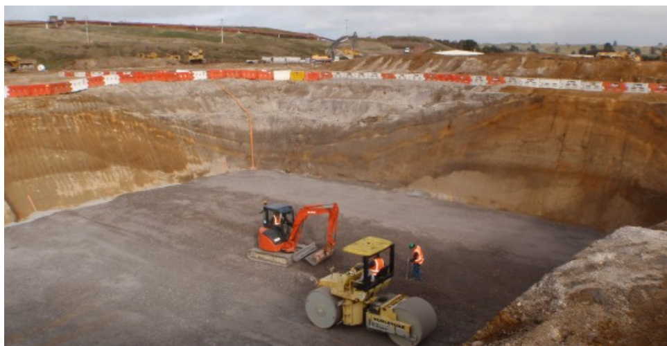
Turbine hall exposure.
