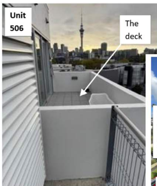
Figure 1: view of deck looking east (prior to the building work)
