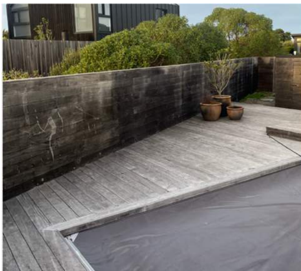
Figure 1: The part of the pool barrier along the southeast boundary 1
