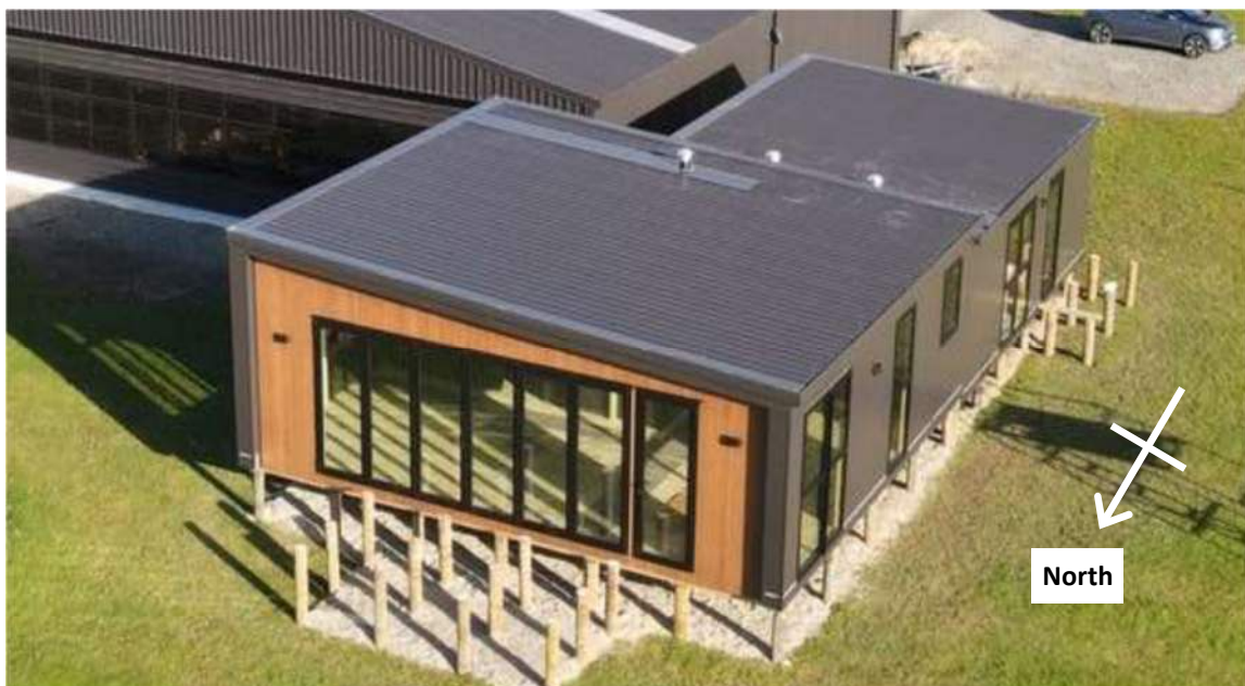
Figure 1: Aerial photo of the modular dwelling (in foreground), on-site in Mandeville.
