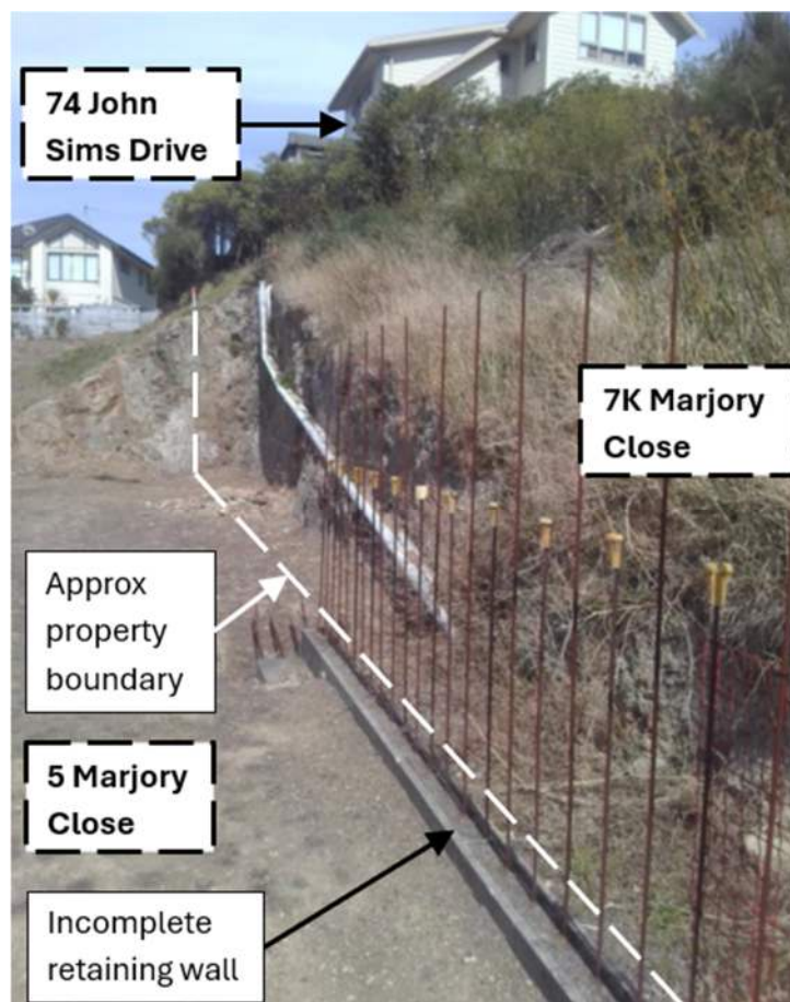
Figure 1: View of neighbouring properties looking south
