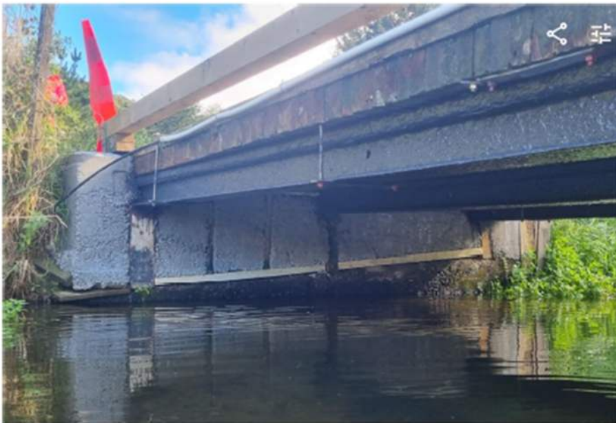
Figure 2: Photo of the bridge and true left abutment following repair.
