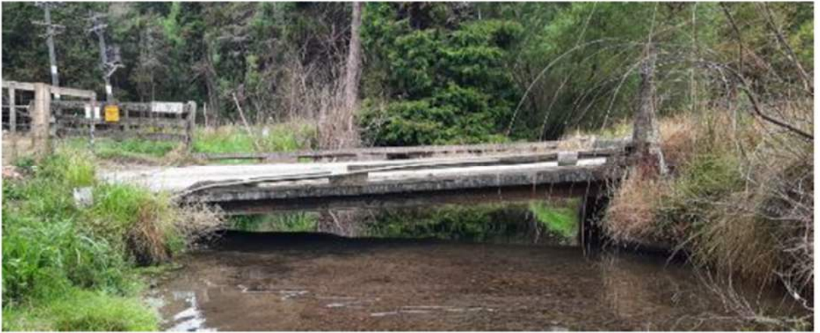
Figure 1: Photo of the bridge prior to the flooding and subsequent repair.
