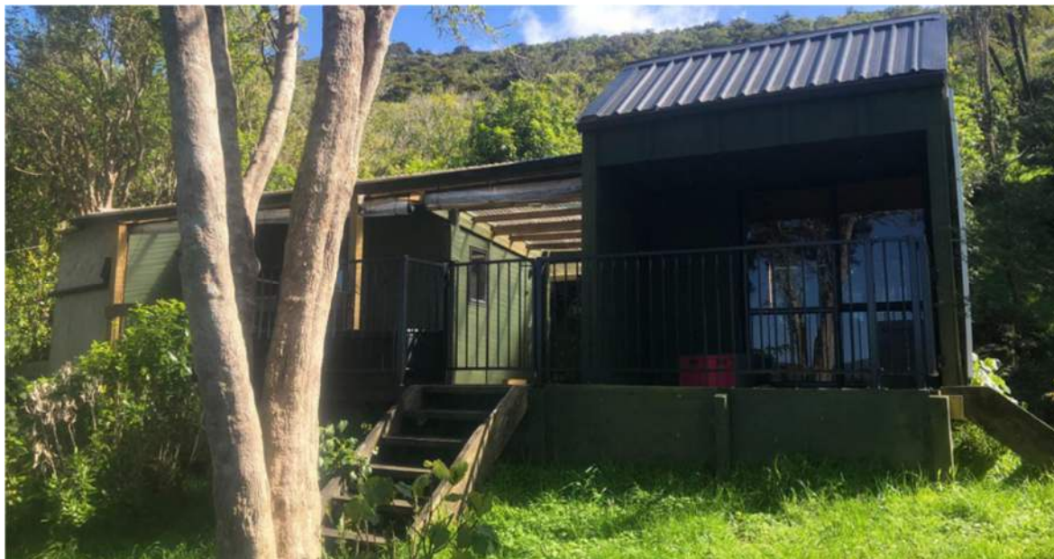
Figure 1: photo of the building work, dated 10 September 2025
