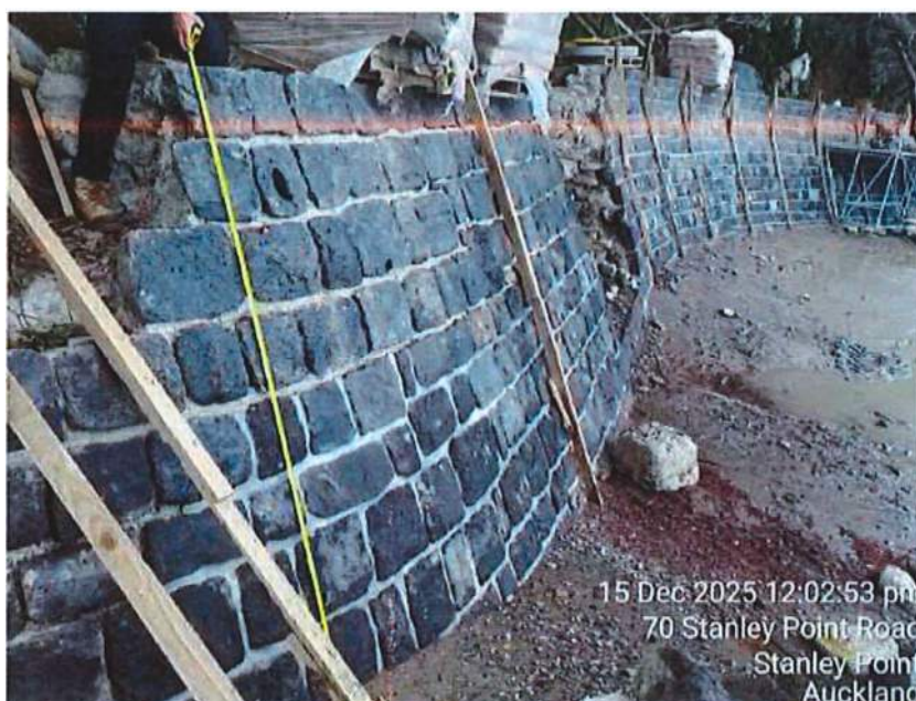
Figure 1: the seawall in Dec 2025, during construction
