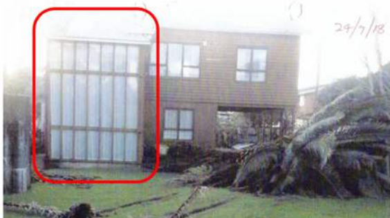
Figure 12: Photo showing the previous stairwell area (dated 24 July 2018).
