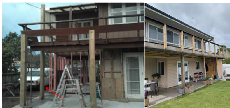
Figure 10: The former deck construction (left) and current deck construction (right).
