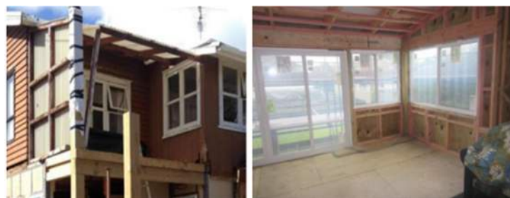
Figure 6: Photos of the former first-floor deck area (left) and current extension of lounge (right).
