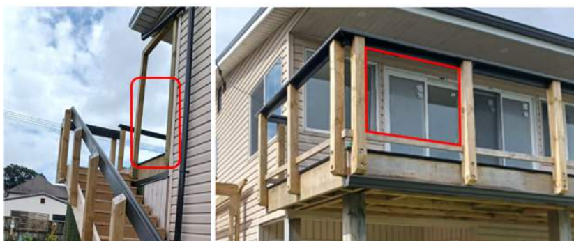
Figure 3: Photos indicating the area without a barrier (left) and the open spaces between the posts and rails (right), taken 16 October 2023.
