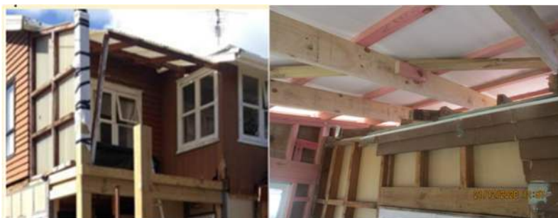
Figure 7: The former first-floor deck (left) and the roof alteration (right).
