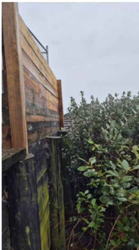
Figure 1: Photo of the timber fence on top of the retaining wall (photo taken from neighbouring property).
