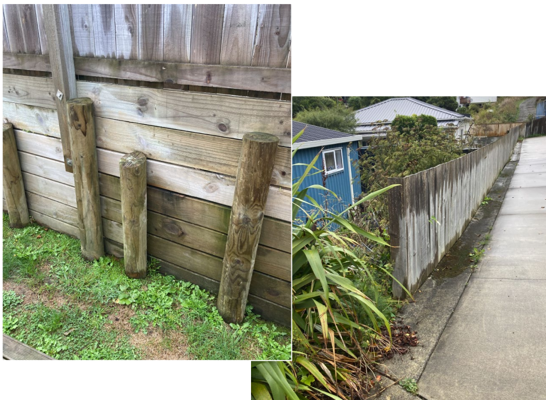
Figure 1: The retaining wall (left) and surface water management system (right)
