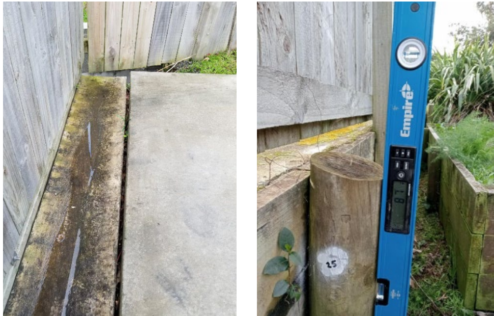
Figure 5: Separation of the dish channel of the surface water management system (left) and leaning posts (right)
