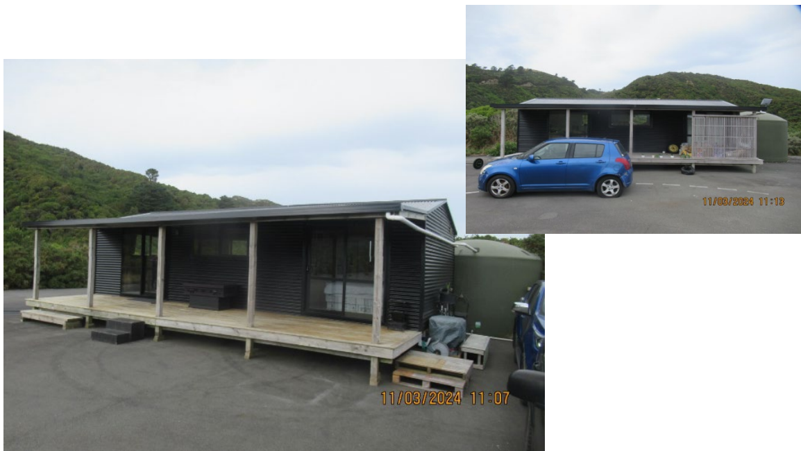
Figure 1: Photos of the two units taken during the authority's inspection
