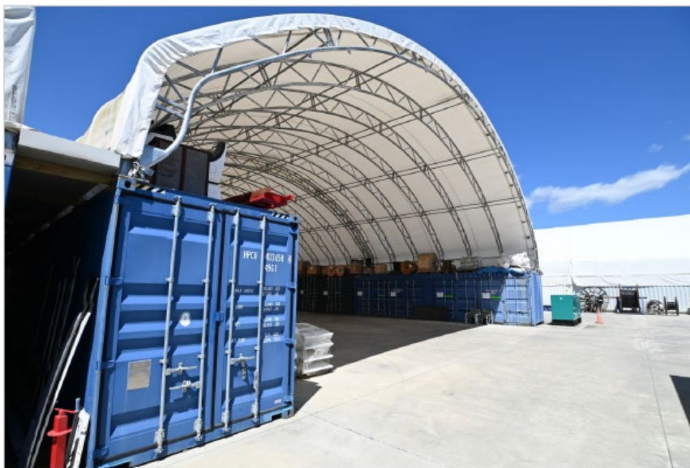
Figure 1. One of the container and canopy structures (structure 3).
