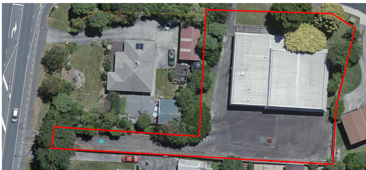
Figure 1: Aerial view of telecommunications exchange structure (property boundary in red)
