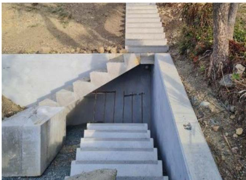
Figure 4: Photo of the upper stairway and elevated landing
