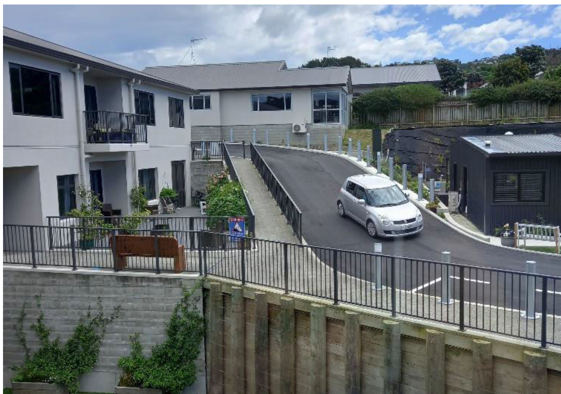
Figure 1: Photograph showing the sloped walkway
