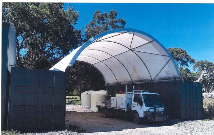
Figure 1: Photograph of the container arch structure, taken by the authority on 19 February 2021.
