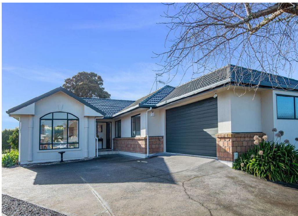
Figure 1: Photograph of the dwelling
