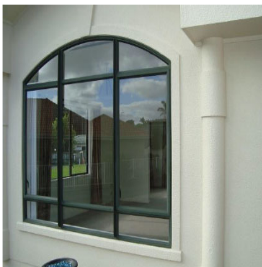
Figure 3: Curved lounge window
