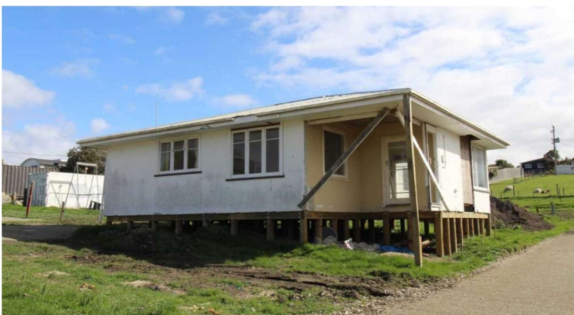
Figure 3: Photograph of the dwelling following relocation.
