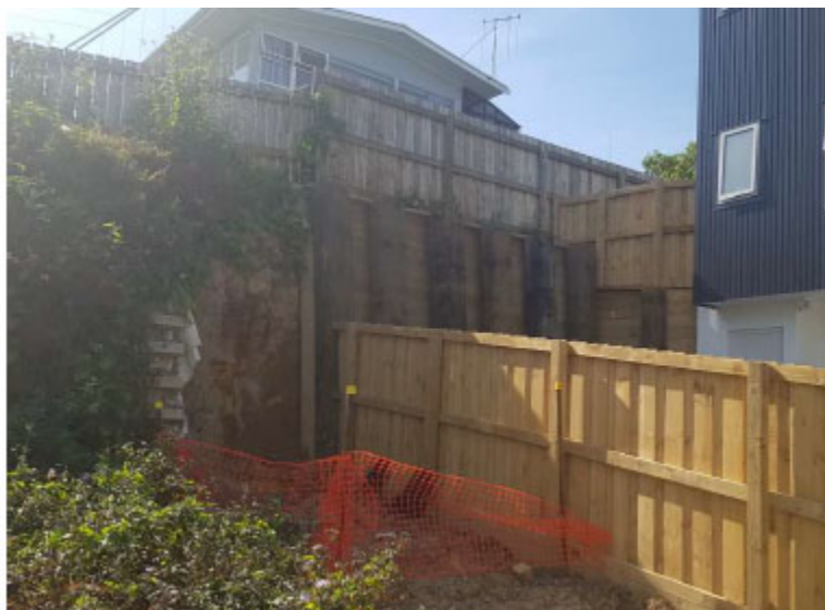
Figure 1: Photograph of unretained cut 1
