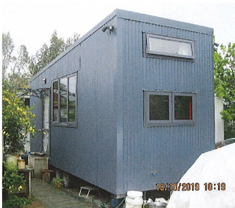
Figure 1: Photograph of the unit on the property
