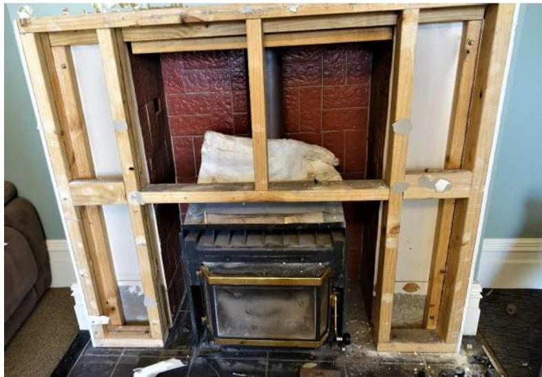
**Figure 1: Photograph of the as-built woodburner**
