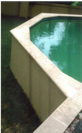
Figure 3: the edge of the swimming pool wall
