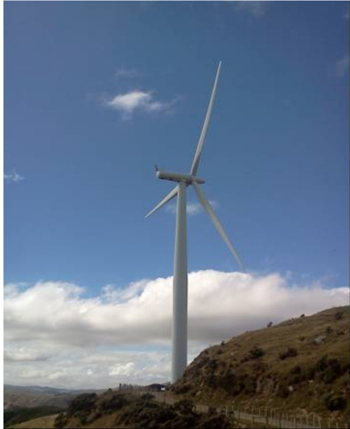
Photo 2 and 3: Completed turbine and base under construction
