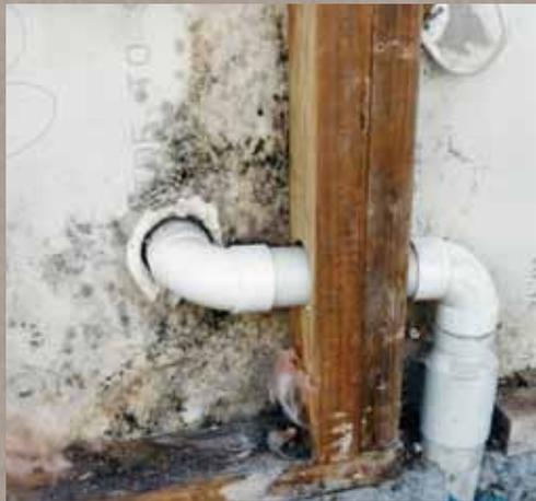
6. Mould on plasterboard lining around a leak
