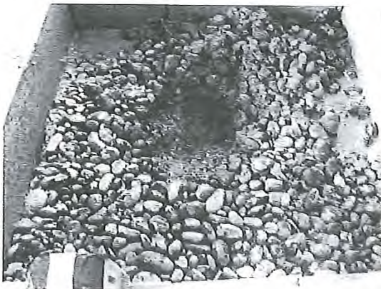
Hardfill contamination [redacted] garage)
