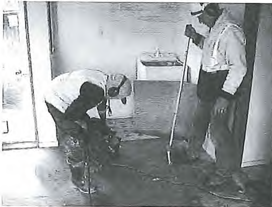
Cutting the garage floor [redacted]
