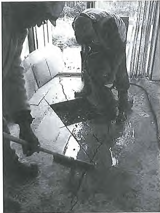
Cutting second panel (dining area)
