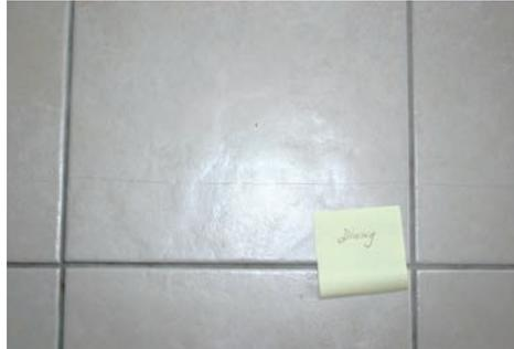
Random cracks in the floor slab which reduce in width to close to indiscernible as they approach the perimeter foundation (or any internal foundation) are shrinkage cracks and are not caused by an earthquake.
