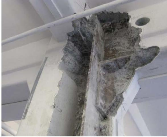
**Figure C6.1: A typical riveted beam-column connection**
