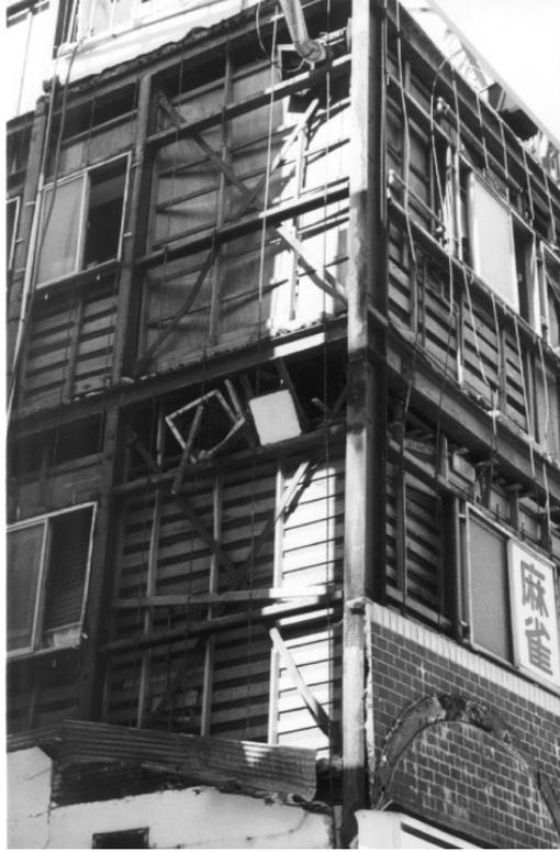
**Figure C6A.4: Braced frame with light tension bracing showing damage but no collapse from the 1995 Kobe earthquake**
