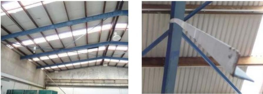
**Figure C6.7: Roof bracing that failed during the February 22, 2011 Christchurch earthquake (Clifton and El Sarraf, 2011)**
