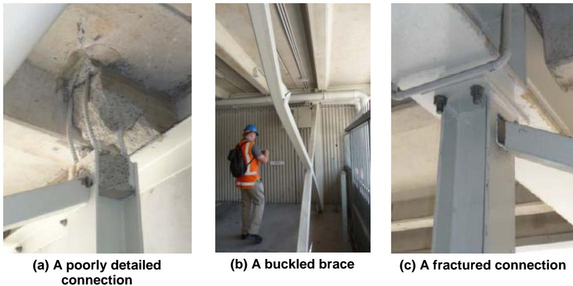
**Figure C6.5: Damaged CBFs in a single-storey car park building during the February 22, 2011 Christchurch earthquake (Clifton and El Sarraf, 2011)**
