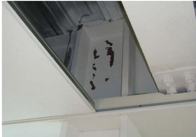
Figure C6.3: Panel zone of an MRF showing minor inelastic action (Clifton and El Sarraf, 2011)
