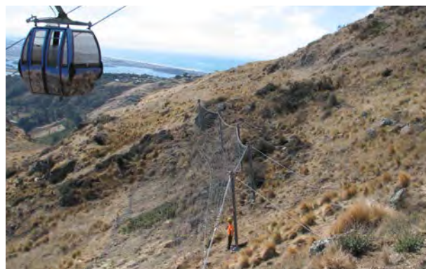
Figure 14: Rockfall attenuator system at Diana Falls (photo Geovert)
