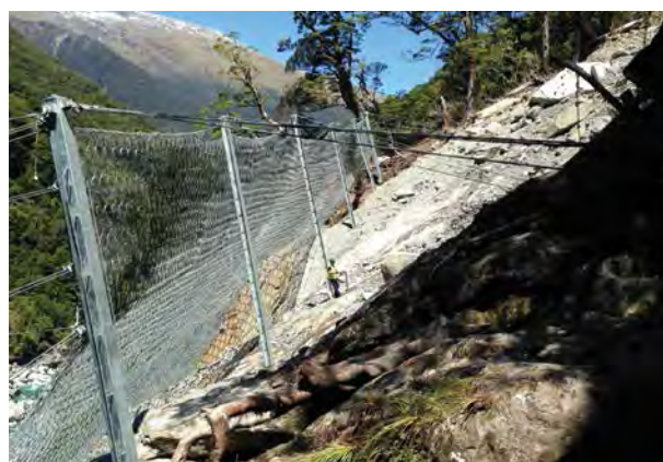
Figure 14: Rockfall attenuator system at Diana Falls (photo Geovert)
