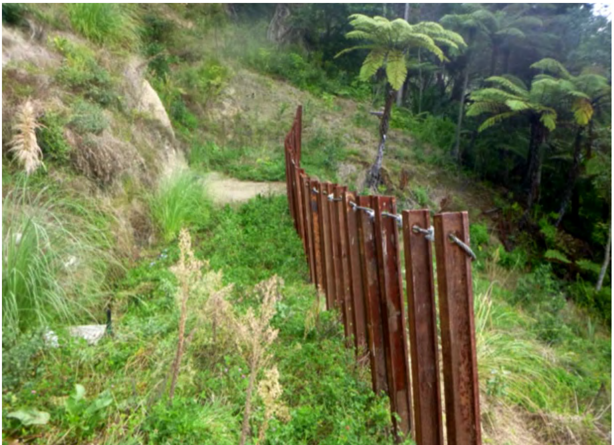
Figure 11: Flexible rockfall barrier (driven railway irons plus cable connection)
