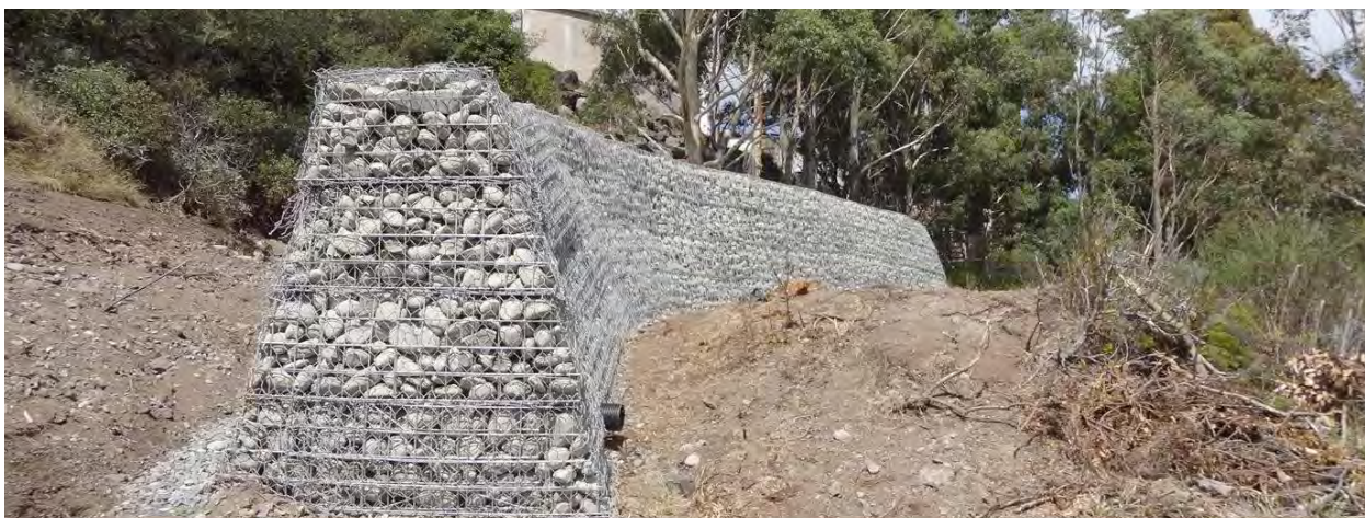
Figure 7b: Mechanically stabilised earthbund rockfall barrier
