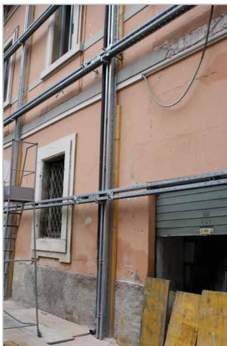
**Figure 30:** L'Aquila, Italy October 2011. Cold-formed steel channel waling and soldiers with threaded rod transverse ties. Note: this type of temporary work can encroach onto footpaths and road corridors, which can be an issue if there is limited space. (Photo: Win Clark)
