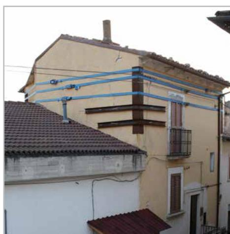
**Figure 32:** L'Aquila, Italy October 2011. Heavy-duty polyester webbing ratchet straps fitted around the building perimeter. Note steel angle plate to protect the straps, and distribute the clamping load into the corner masonry. (Photo: Win Clark)
