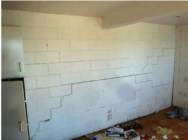
**Figure A.2: Damaged concrete block basement wall**
