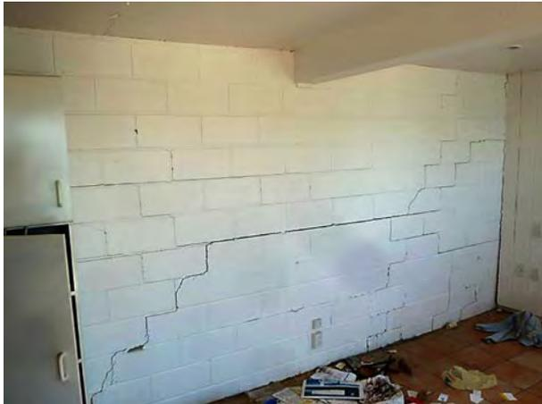
**Figure A.2: Damaged concrete block basement wall**
