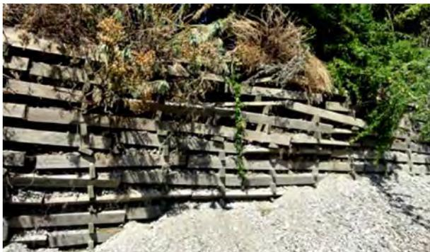
**Figure A.4: Damaged timber crib wall**
