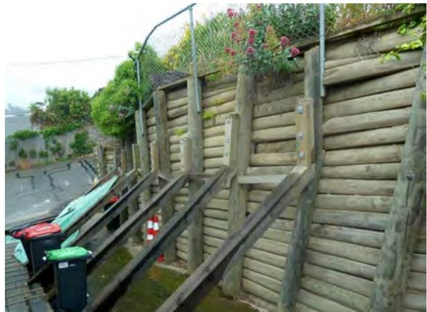
**Figure A.3: Damaged timber pole wall showing failure of poles at anchor location and failure of anchors**
