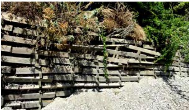
**Figure A.4: Damaged timber crib wall**
