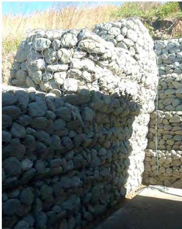
**Figure A.6: Gabion wall showing bulging and outwards movement**
