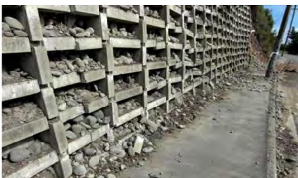
**Figure A.5: Concrete crib wall showing loss of rounded gravel backfill**
