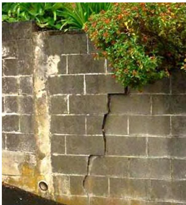
**Figure A.1: Failure of poorly constructed concrete block retaining wall**
