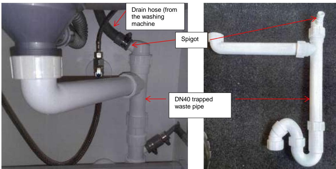
**Figure 1: Photographs of the appliance connections and DN40 trapped waste pipe**
