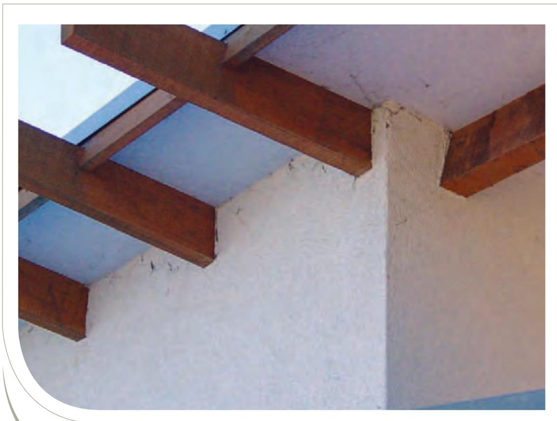
Figure 7.7 Exposed rafters with junctions that are difficult to weatherproof.
