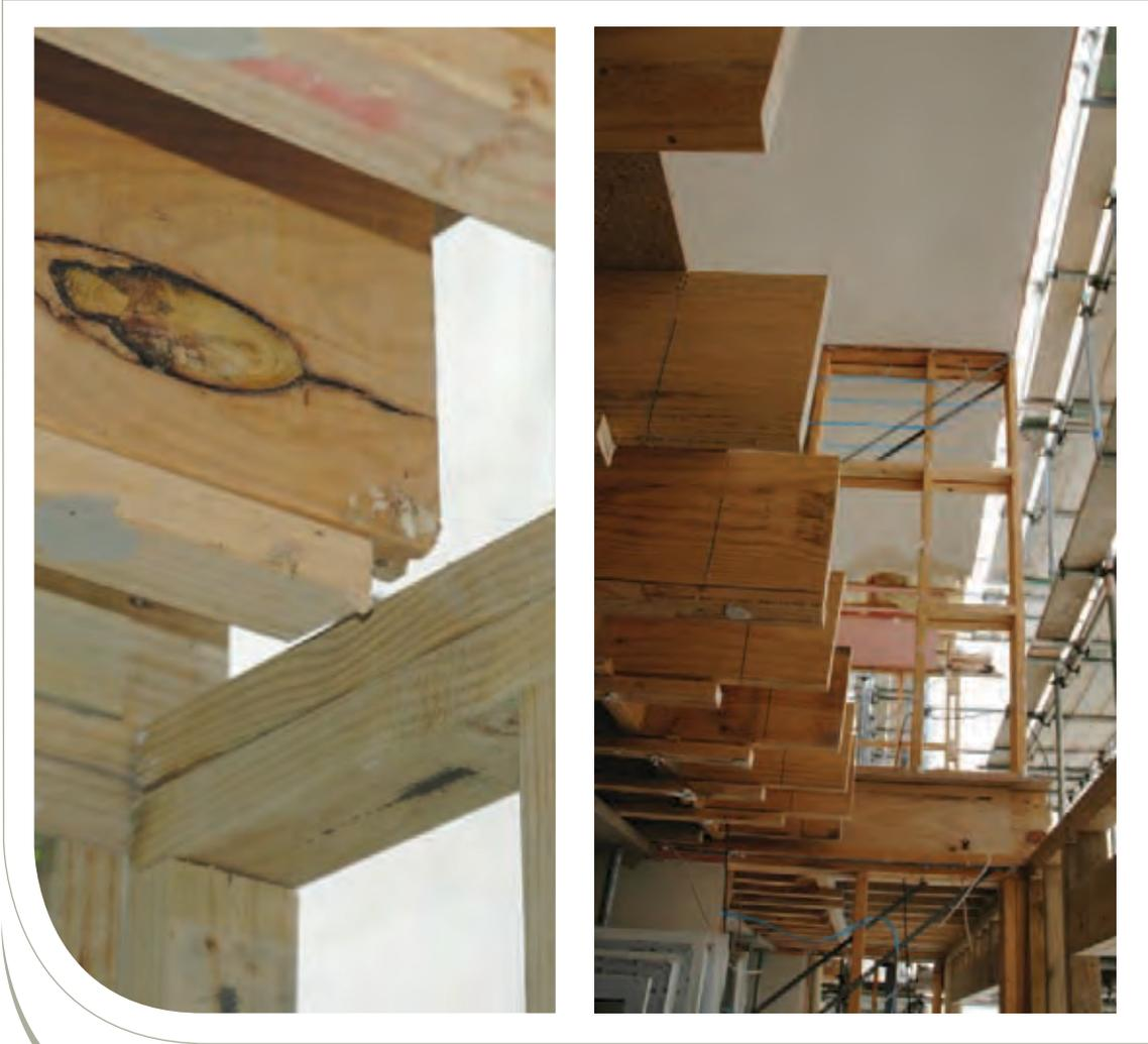
Figure 6.2 Two photos showing the difference in extent of floor joist removal in adjacent units in the same complex.
