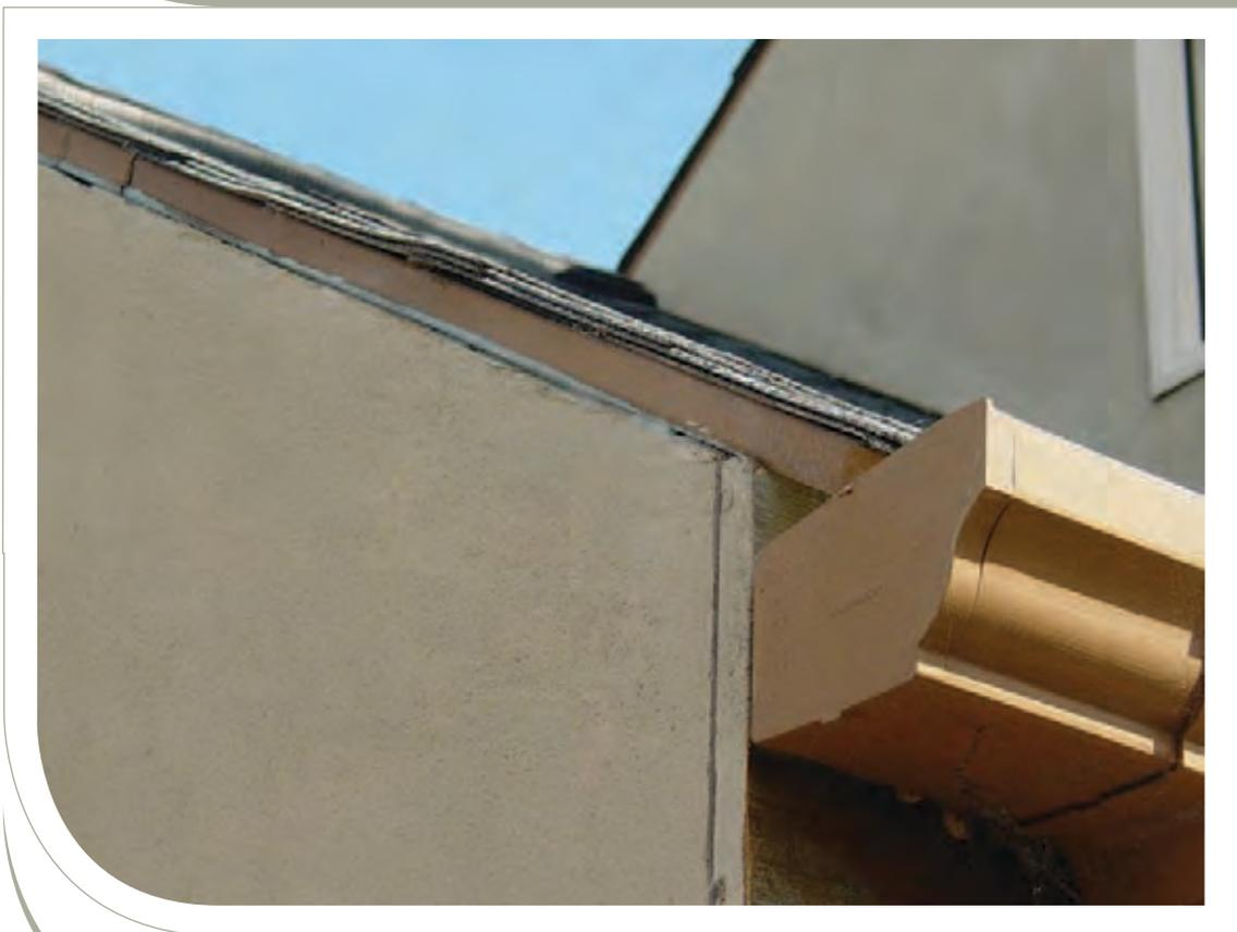
Figure 7.9 Stucco cladding is vulnerable when butted up to blocking along the raking gable end of the building.
