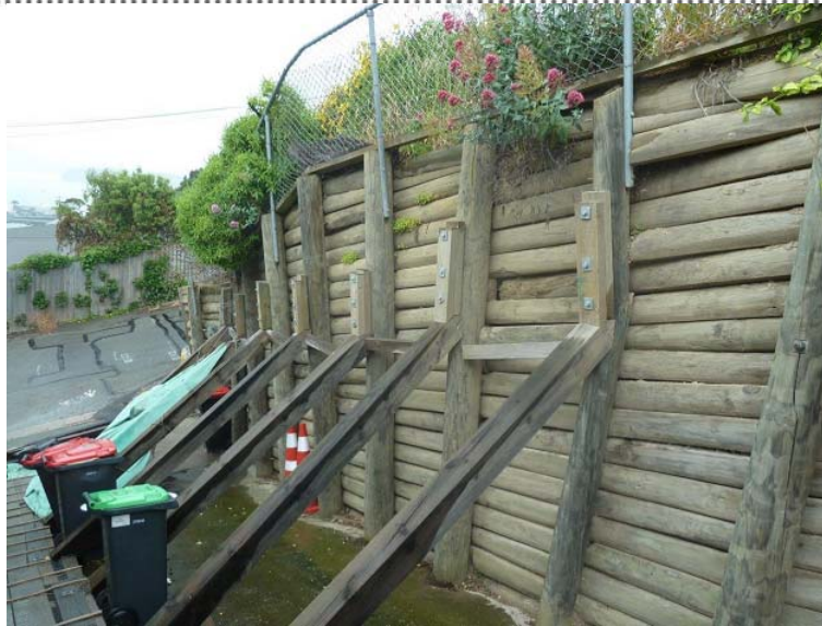
Figure 3: Damaged timber pole wall showing failure of poles at anchor location and failure of anchors
