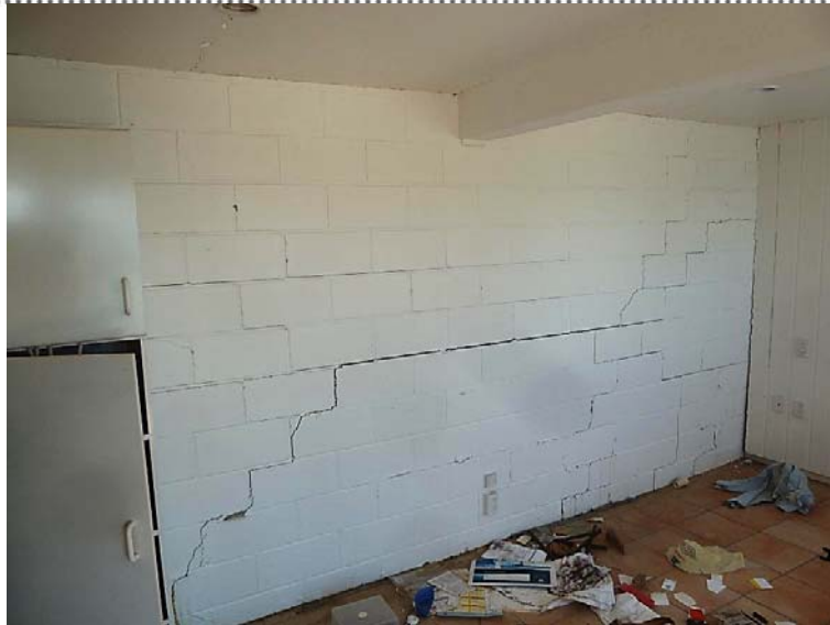
Figure 2: Damaged concrete block basement wall
