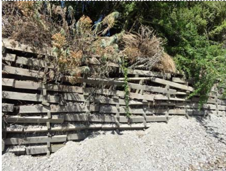
Figure 4: Damaged timber crib wall
