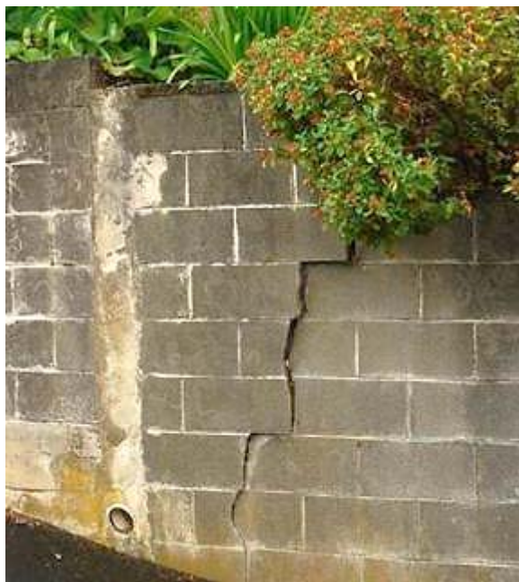
Figure 1: Failure of poorly constructed concrete block retaining wall
