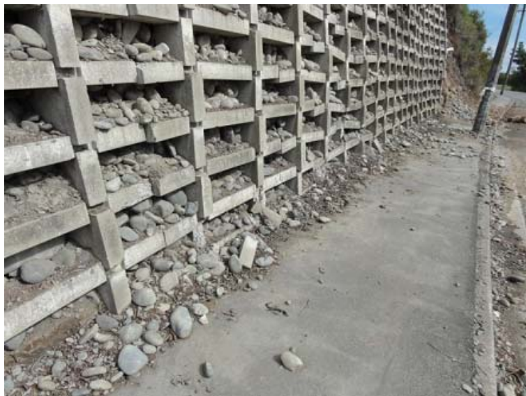
Figure 5: Concrete crib wall showing loss of rounded gravel backfill
