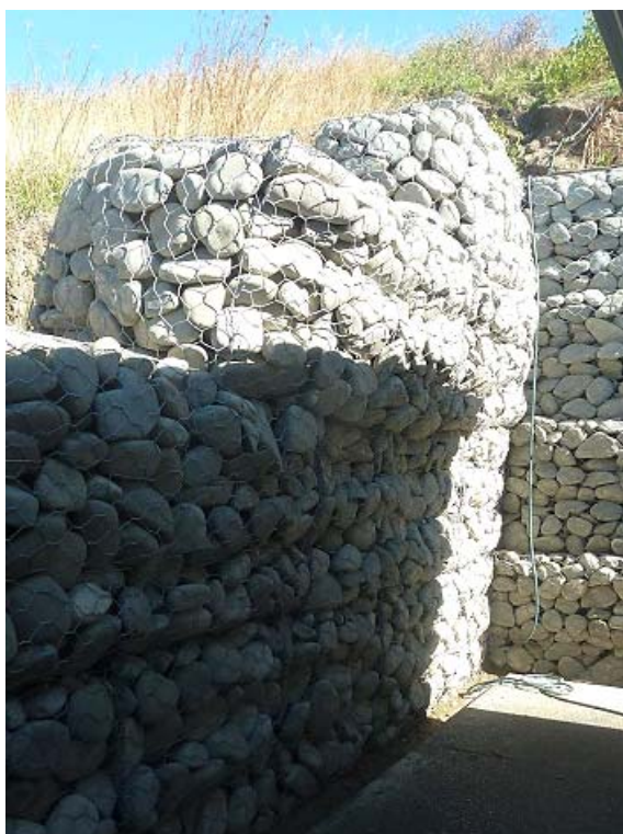
Figure 6: Gabion wall showing bulging and outwards movement
