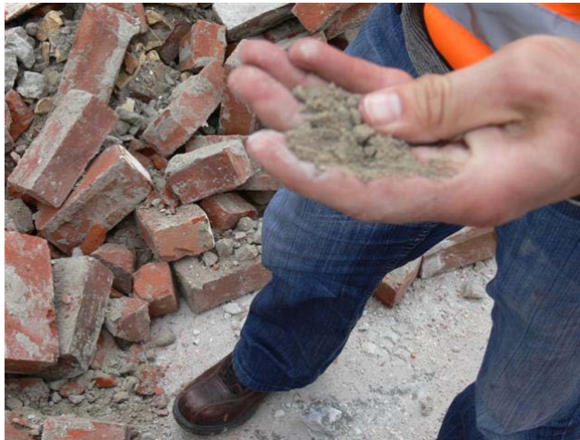
Figure C8.10: Soft mortar. Note the delaminated mortar from bricks in the background. (Ingham and Griffith, 2011)
