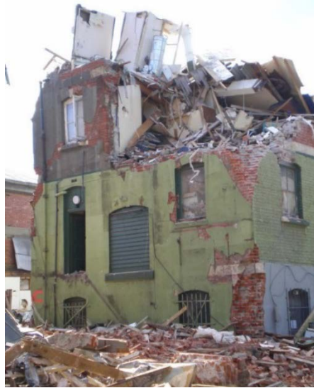
Figure C8.30: Reduction of damage towards base of building as axial load increases (Dunning Thornton)
