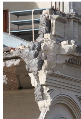
(c) Stone facing and concrete core
