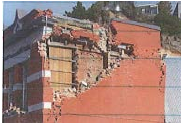
(c) Post-June 2011 event – wall collapse
