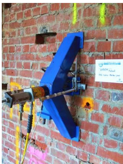
(a) Typical anchor pull test set-up
