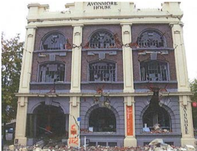
Figure C8.46: Failure of spandrels. Also note rocking of upper piers and corner cracking of the parapet. (Dizhur)
