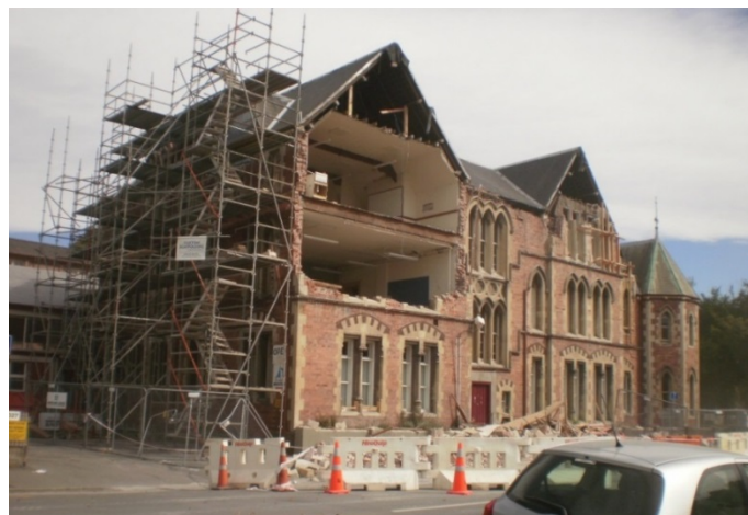
Figure C8.14: A lack of connection of the walls parallel to joist and rafters with diaphragms and return walls leading to collapse of wall under face load
