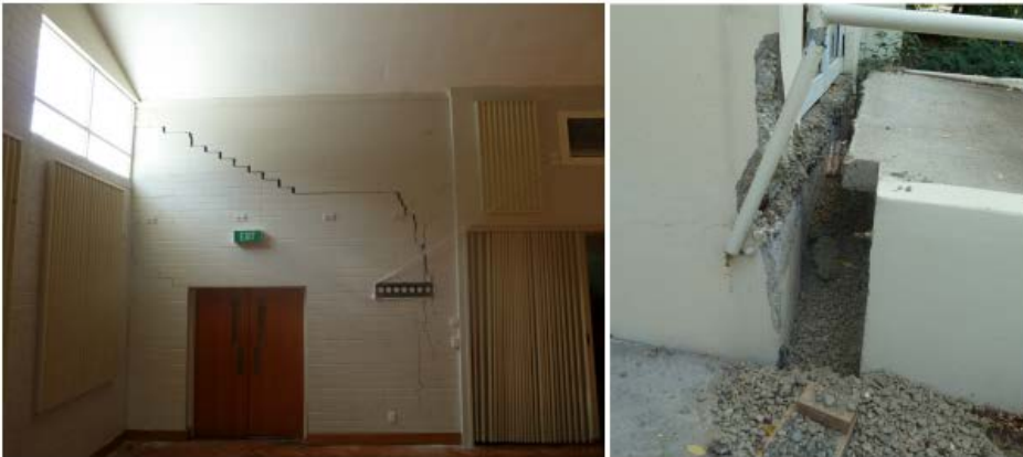
(a) Large diagonal cracks and lateral movement of the access ramp caused by ground movement
