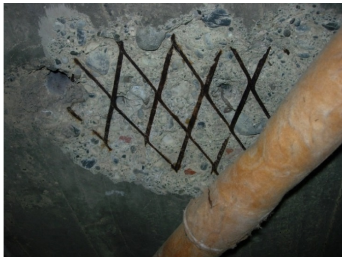
Figure C8.11: Concrete slab with expanded metal lath reinforcement. Corrosion of the lath from carbonation of the concrete over time has caused the concrete to spall.
