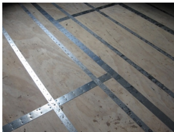
Figure C8.25: New plywood diaphragm (Holmes Consulting Group)
