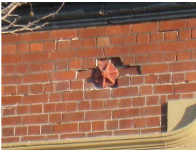
Figure C8.34: Plate anchor on verge of punching shear failure (Dizhur et al., 2011)
