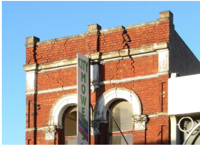
Figure C8.21: The wide cracks through bond beams indicate a lack of reinforcement in the beam (Dizhur)
