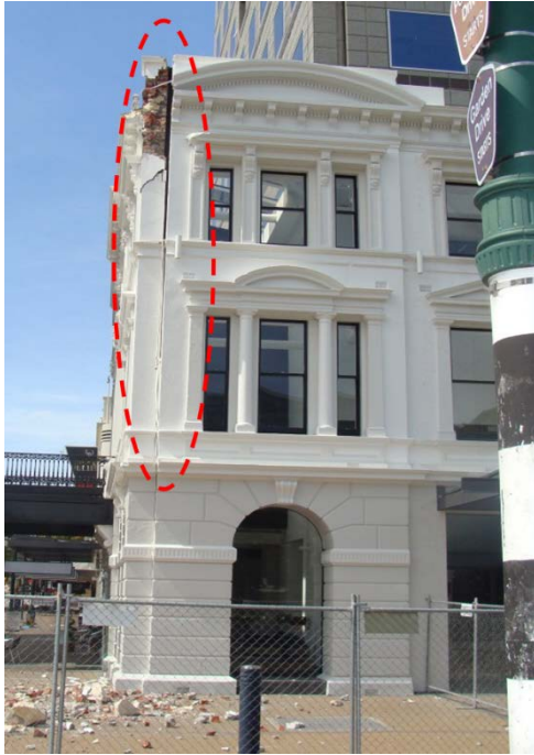
(a) Vertical cracks (Dizhur)
