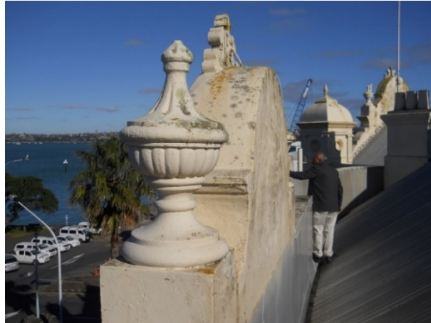
Figure C8.22: Secondary elements (Miyamoto International)
