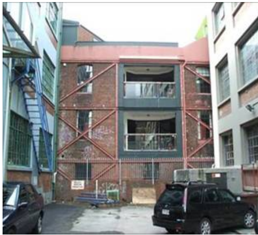
(a) Concentric steel frame (Beca)
