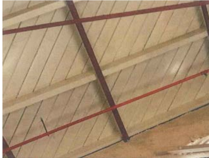
Figure C8.13: Typical timber diaphragms – diagonal sarking
