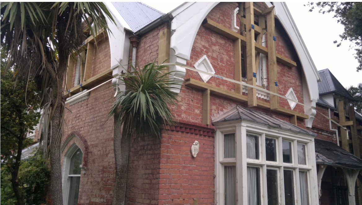
Figure C8.1: Temporary securing of a mildly damaged solid masonry URM building (Dunning Thornton/Heartwood Community)
