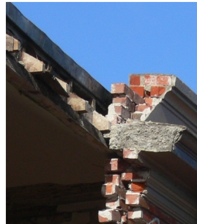
(b) Roof seating arrangement and parapet wall (Dymtro Dizhur)
