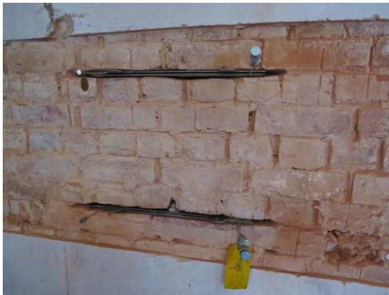
(a) Cutting mortar bed-joints and insertion of flat jacks into clay brick masonry
