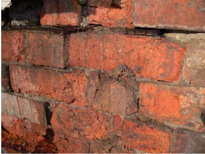
Figure C8.52: Severely degraded bricks and mortar due to moisture ingress (Ingham and Griffith, 2011)
