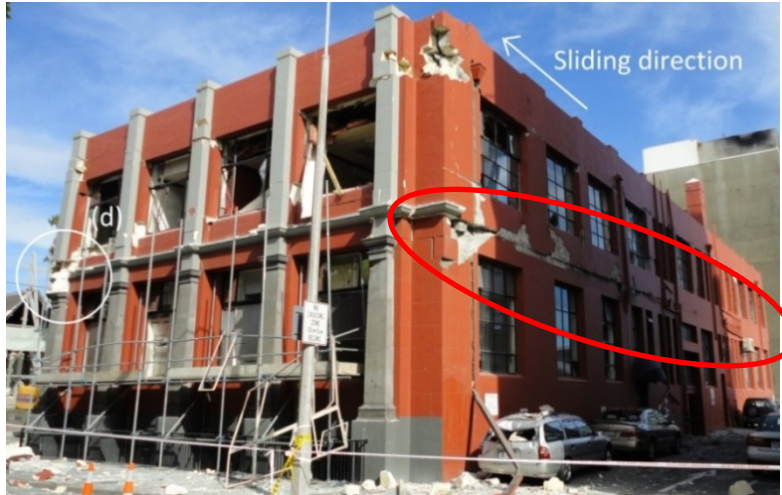
(a) Sliding shear failure along a defined plane at first floor level (Dunning Thornton)
