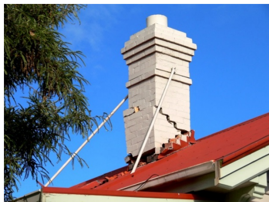
(b) Chimney at onset of falling (Dizhur)
