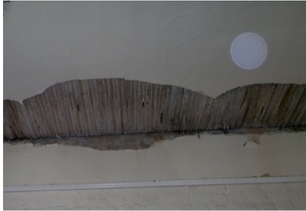
Figure C8.32: Lath and plaster ceiling. Note that stresses where shears are transmitted to the wall have caused the plaster to delaminate from the timber lath.
