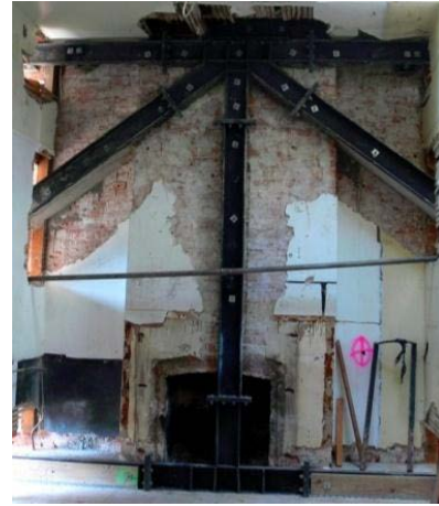
(b) Steel frame (Dizhur)
