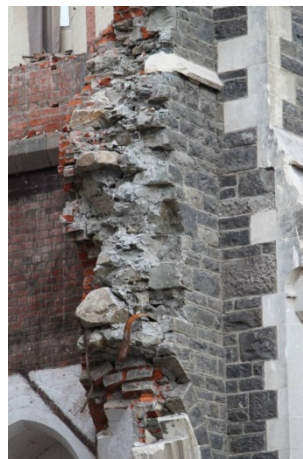
(b) Stone facing and brickwork backing
