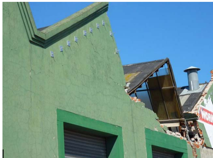
Figure C8.40: Collapse of gable wall. Note a secured gable end that survived earthquake loading and a companion failed gable end that was not secured. (Ingham and Griffith, 2011)
