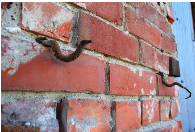
Figure C8.53: Metal cavity ties in rusted condition (Dizhur et al., 2011)
