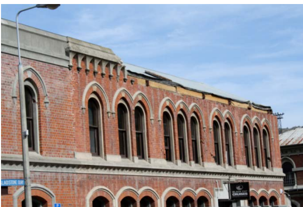
(a) Out-of-plane instability of parapet (Beca)
