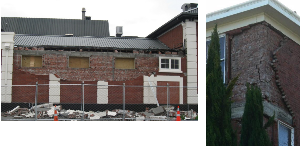
Figure C8.41: Failure of URM cavity walls (Dizhur)
