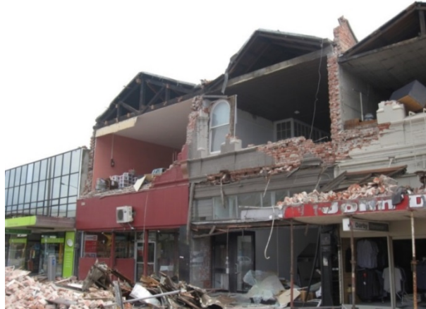
Figure C8.48: Face-load failure of URM façade exacerbated by outward loadings from downward force on canopy. Note the adjacent propped canopy did not collapse. (Dunning Thornton)
