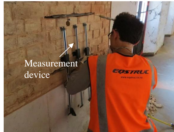
(b) In situ deformability test set-up under preparation in clay brick masonry
