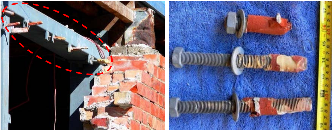
Figure C8.37: Failed adhesive brick anchors (Dizhur et al., 2013)
