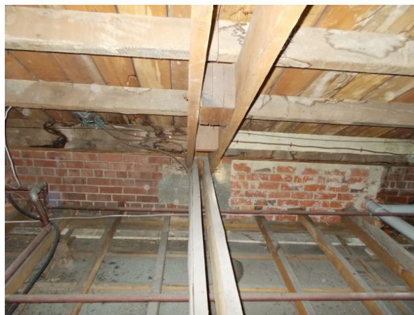
(c) Wall to roof truss connection. Note truss is seated on a concrete padstone (Miyamoto International)
