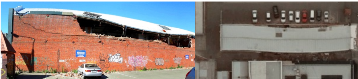
Figure C8.31: Out-of-plane wall failure due to excessive roof diaphragm movement (Dizhur et al., 2011)
