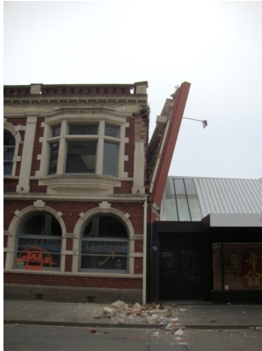
Figure C8.39: Out-of-plane instability of wall under face load due to a lack of ties between the face-loaded wall and the rest of the structure (Sharpe)
