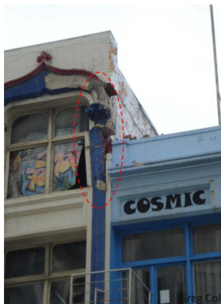
Figure C8.49: Pounding failure (Cole)
