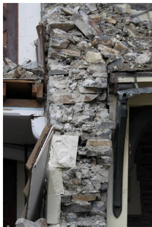
(a) Dressed stone in outer leaves and “rubble” fill
