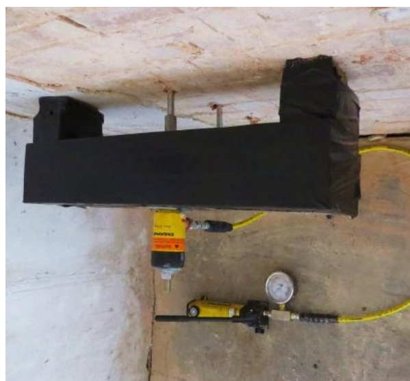
(b) Close up of the typical test set-up with an alternative test frame
