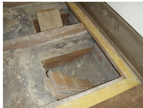
(b) Floor joist to wall connection. Note presence of steel strap (Matt Williams)
