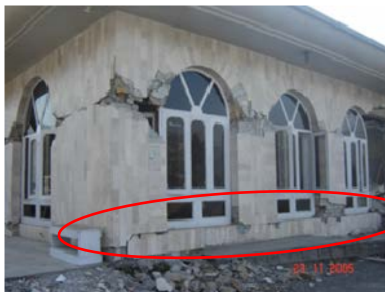
Figure C8.43: Rocking and delamination of bricks of a one-storey unreinforced brick masonry building with reinforced concrete roof slab (Bothara and Hiçyılmaz, 2008)
