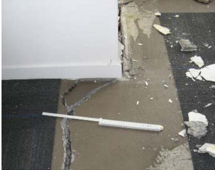
**Figure C5.19: Observed separation between floor and supporting beam due to beam elongation in 2011 Canterbury earthquakes (Bull)**
