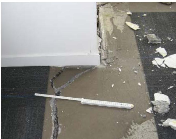
**Figure C5G.4: Observed separation between floor and supporting beam due to frame elongation in 2011 Canterbury earthquakes (Des Bull)**
