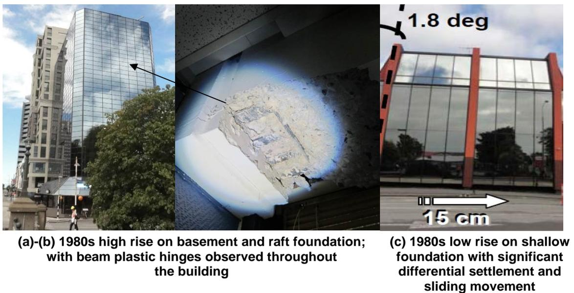
**Figure C4D.3: Building foundation “failure” (Cubrinovski and McCahon, 2012)**
